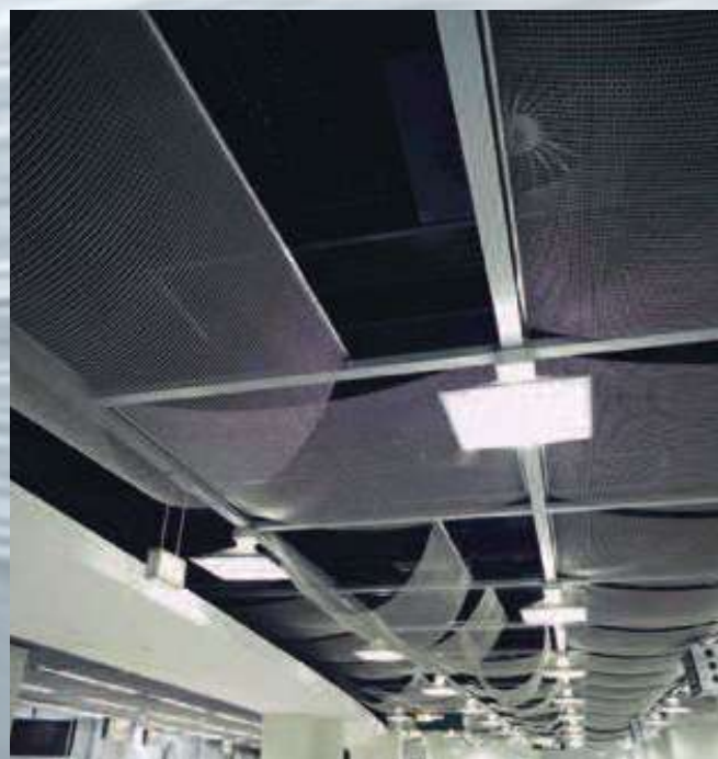
Adjustable mounting system for ceilings with sag.
