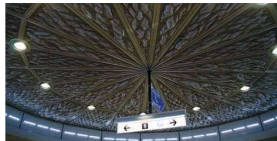
Three-dimensional stainless-steel mesh for improving the space's acoustics. Cologne light railway, Germany, MONTANA.
