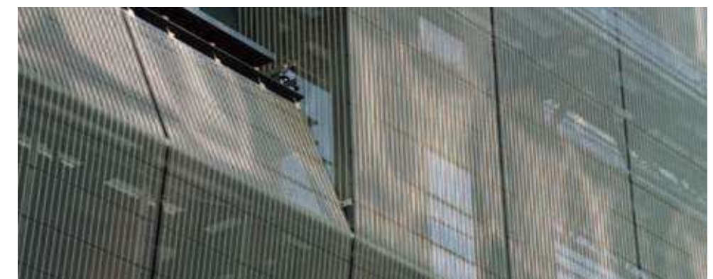
Multidimensional facade with mesh elements deflected by 19°. Júlia Center, Andorra la Vella, Andorra, EGLA-DUO 4212.
