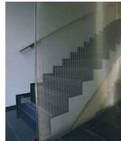
Fall protection on the stairwell with wire mesh cladding made of MULTI-BARRETTE.
