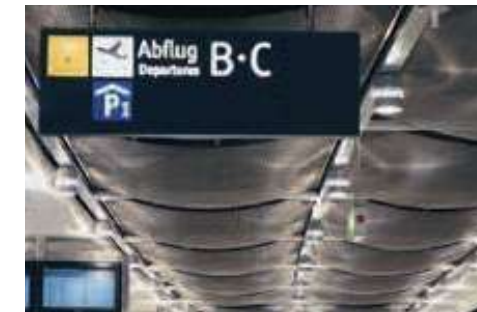
Ceiling elements with sag. Terminal B, Düsseldorf Airport, Germany, DOKAWELL-MONO 8965.
