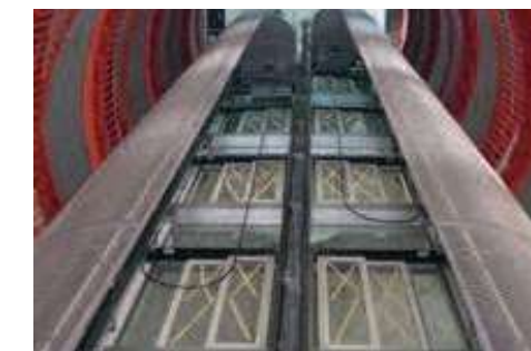
Lift shaft cladding with architectural mesh, Ulm Town Library, Germany, EGLA-TWIN 4243.
