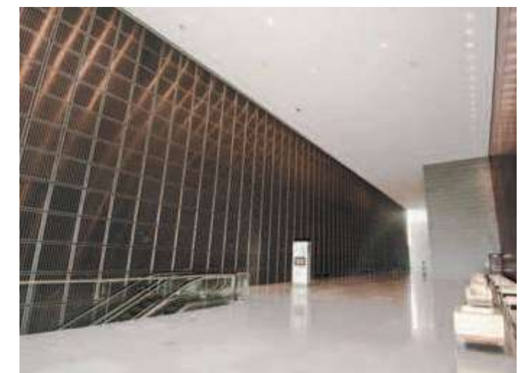
Wire mesh cassettes made of architectural mesh MULTI-BARRETTE 8123. Qatar National Convention Centre, Doha, Qatar.
