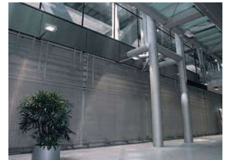
Cladding of technical systems. Terminal 2, Cologne-Bonn Airport, Germany, MULTI-BARRETTE 8123.
