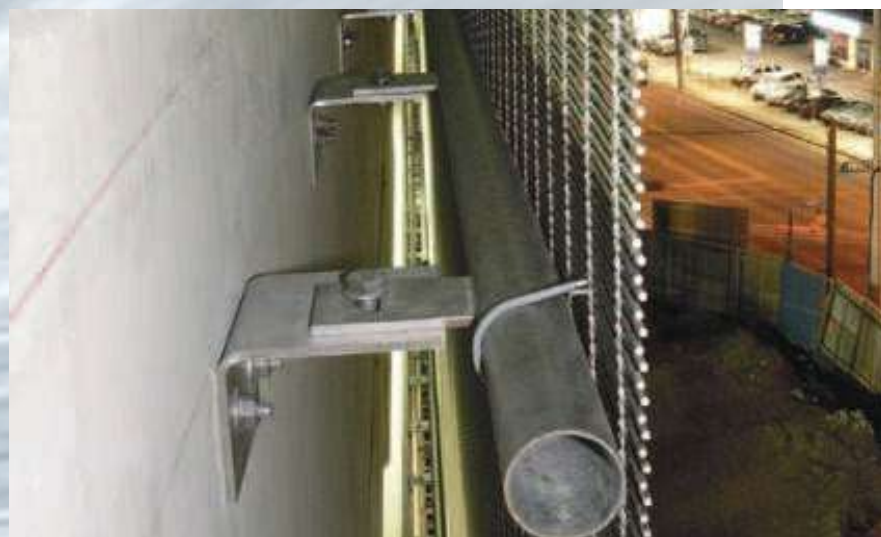
Intermediate mounting: round tube and wire connectors.
