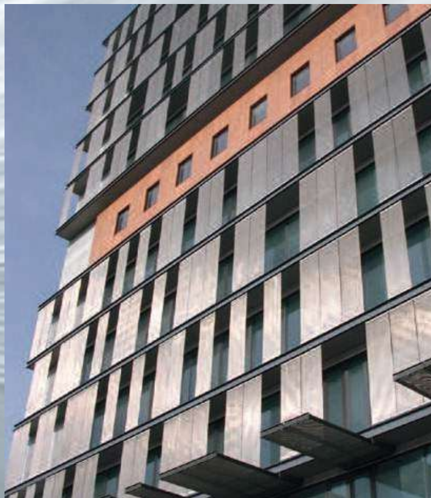
Transparent architectural mesh elements effectively combine sun protection with superb design possibilities. Sun protection facade, Lisbon, Portugal, EGLA-MONO 4391.
