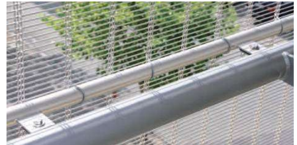
Intermediate mounting: round tube and wire connectors.
