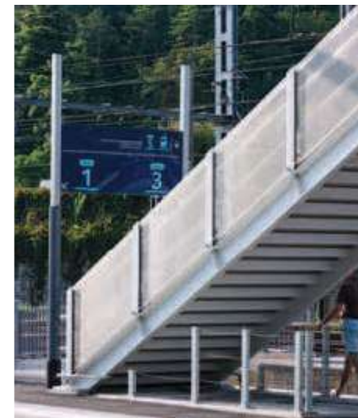
Bridge cladding at a train station made of stainless steel wire mesh EGLA-DUO.
