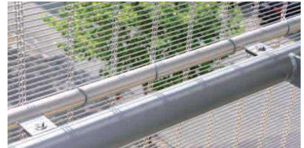
Intermediate mounting: round tube and wire connectors.
