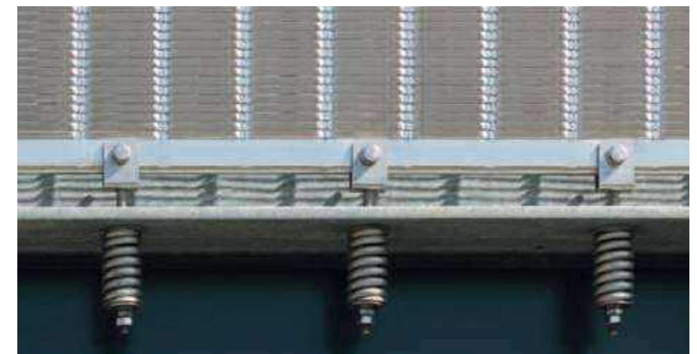
Bottom mounting: flat tension profile, clevis screws and pressure springs.
