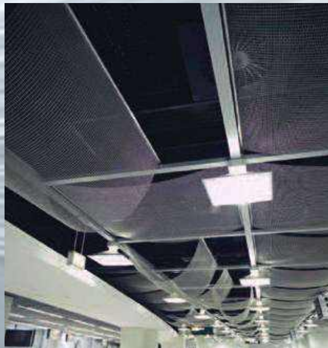
Adjustable mounting system for ceilings with sag.
