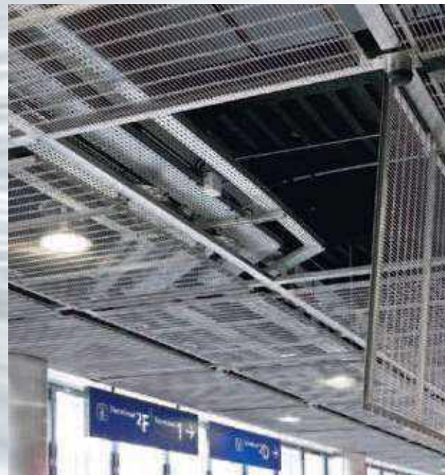
Removable mounting system for ceilings without sag and with framed elements.
