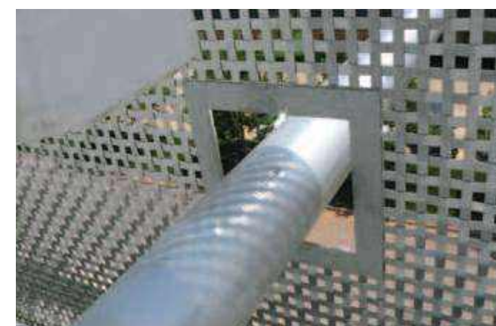
Cut-outs in mesh elements.
